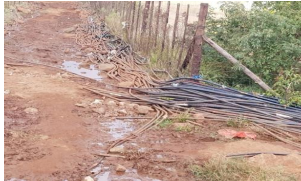
Illegal connections in Raliphaswa village Nzhelele
