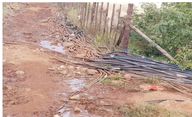
Illegal connections in Raliphaswa village Nzhelele
